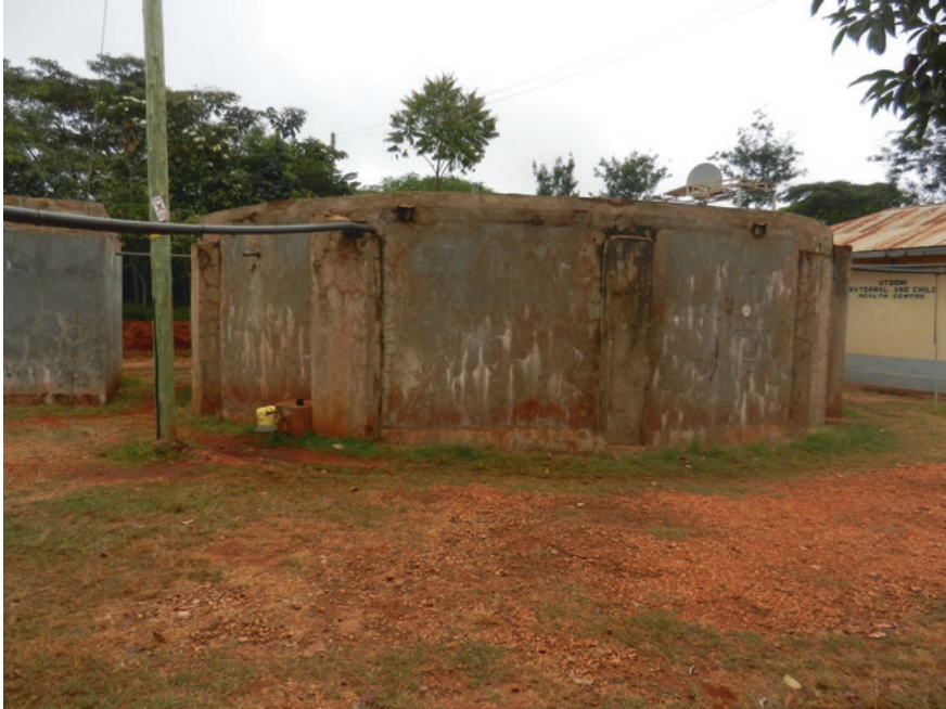
Fig. 2 The UDO compound's main water storage tank, which holds 220,000 liters. The square tank on the left holds 60,000 liters. The main office building is on the right. (Photo by author 2011)
