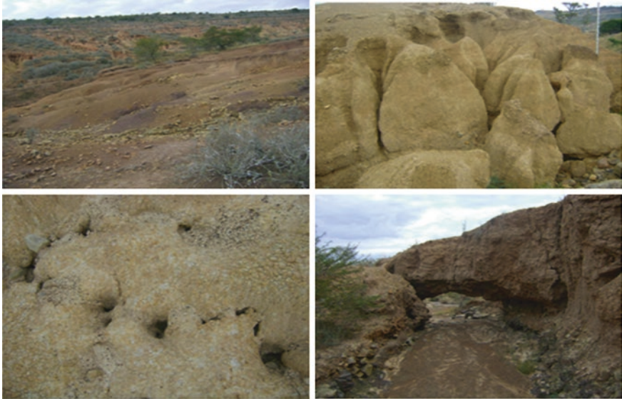
Fig. 6 Piping and gully erosion associated with highly sodic soils derived from mudstones and shales in the Keiskamma catchment, Eastern Cape Province
