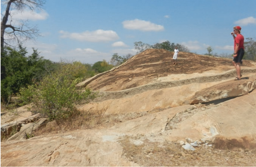
Fig. 3 Catchment area of the Miamba Mitamboni SHG in southern Makueni County. The low cement and rock walls converge at a point behind the shrub in the lower left and feed into a pipe leading to the storage tanks. (Photo by author 2013)
